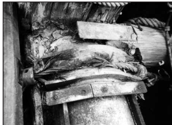
Fig. 33: Saddle of a bridge in an amusement park. Standing water (e.g. trapped on saddles) causes severe local rope corrosion.
