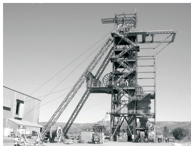
FIG 2 - The P 49 shaft installation: tower.
